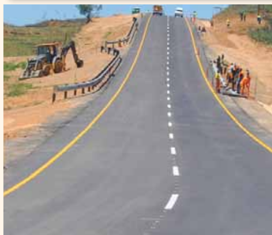
Layer works, Asphalt and Road marking KM 3.400 Widening for final layers & completed intersection of P435 with P522
