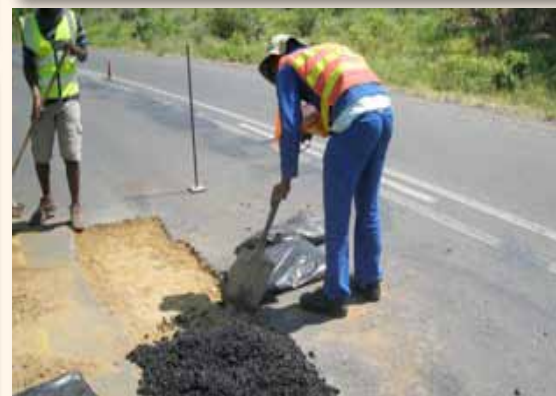
P69 Brick layer roller course 5.8 km & P69 Grade 1 Contractor patching the pothole & erecting Road Signs
