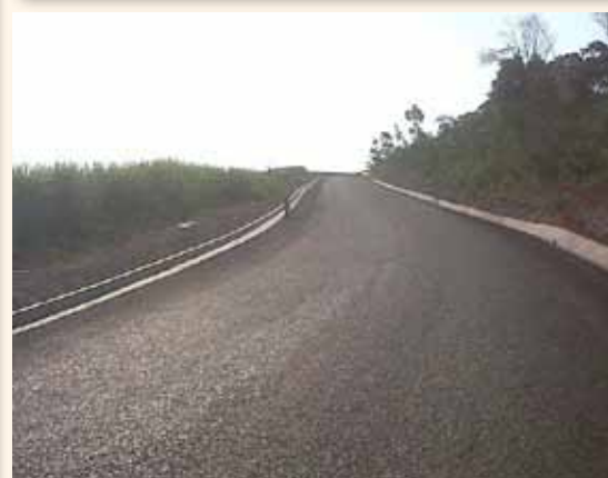
P50-2 Sub-Base, Double Seal surfacing & completed
