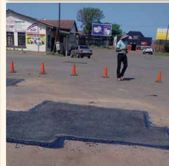
Blacktop patching on P416 & P380 & P2-8 during patching
