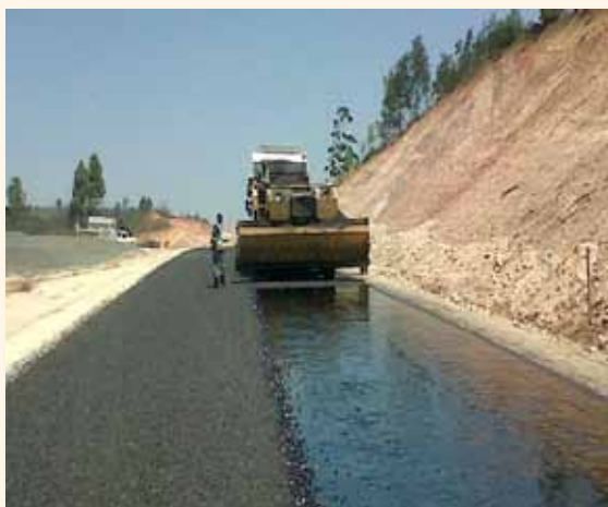
P50-2 Sub-Base, Double Seal surfacing & completed
