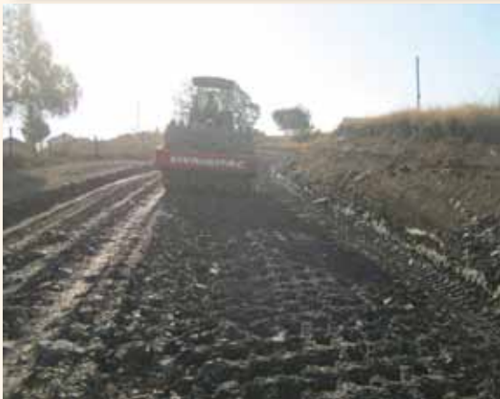
D2421: Processing of the gravel wearing course & D2420: Compaction of gravel wearing course
