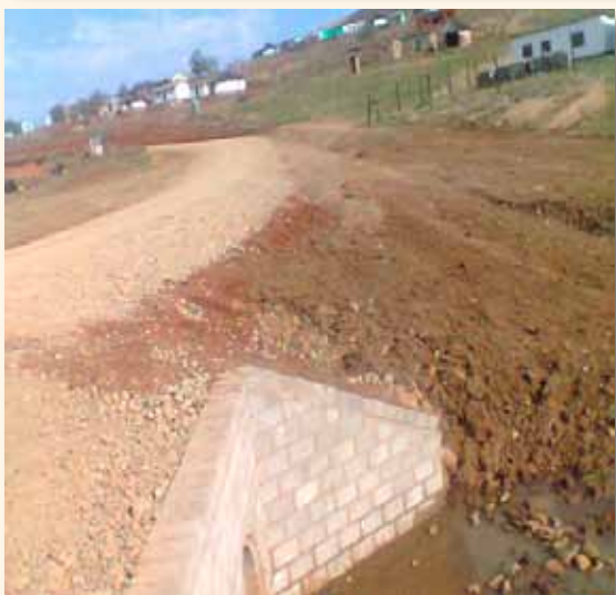
D2416, P129 before & after Betterment and Regravelling Completed on Magcakini Road
