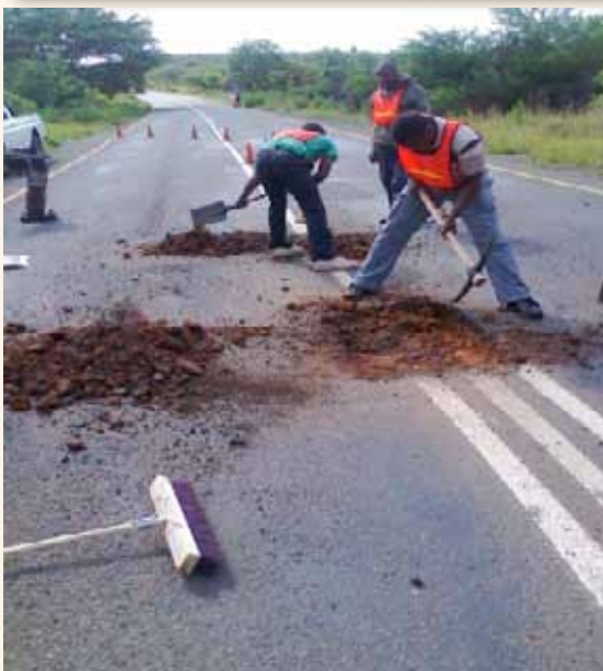
Blacktop patching on P416 & P380 & P2-8 during patching
