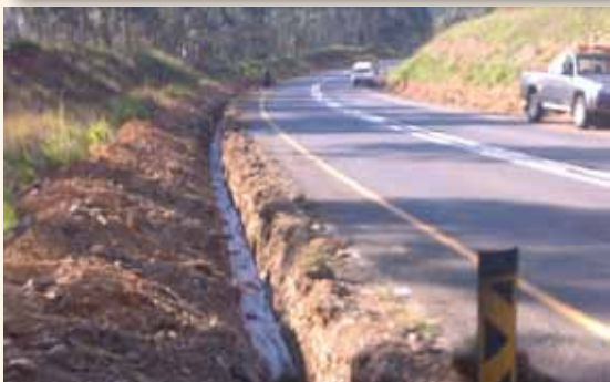
P211 Placing Premix and Constructing Transversal Joint&P356-2 placing, rolling premix KM7.54 & subsoil drainage
