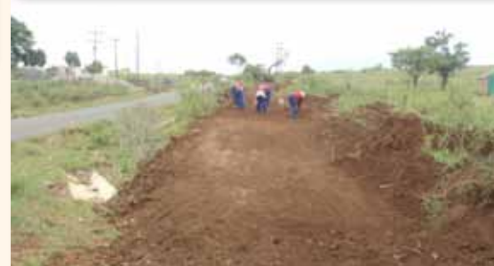
P36-2 Cleaning of inlet & outlet drains & P218 / P710 clearing and grubbing for sidewalks.
