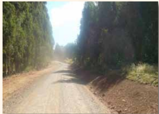
D2421: Processing of the gravel wearing course & D2420: Compaction of gravel wearing course
