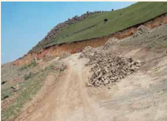
D2421: Processing of the gravel wearing course & D2420: Compaction of gravel wearing course
